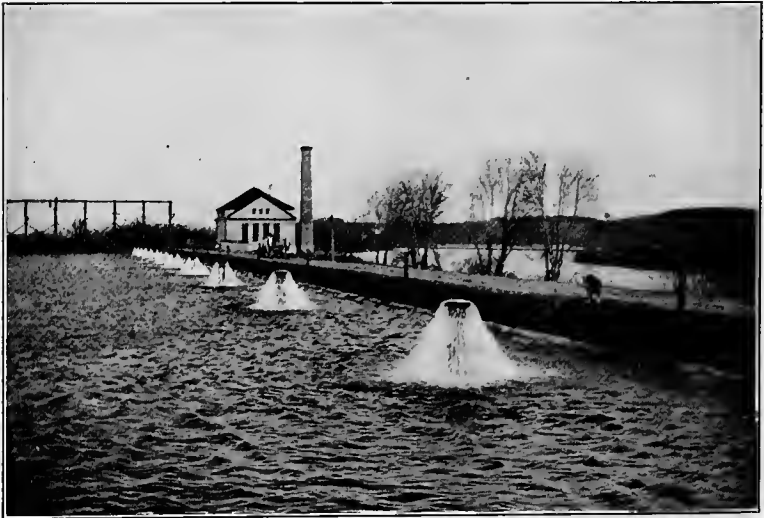
FIG. 64.—Aerators at the Albany Filtration Plant. Designed by Allen Hazen.
