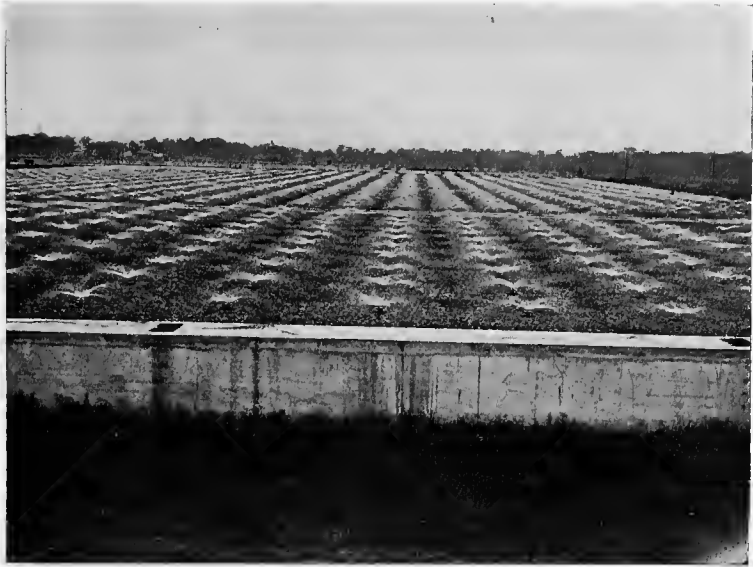
FIG. 65.—Sprinkling Filters, at Baltimore Sewage Disposal Works.
