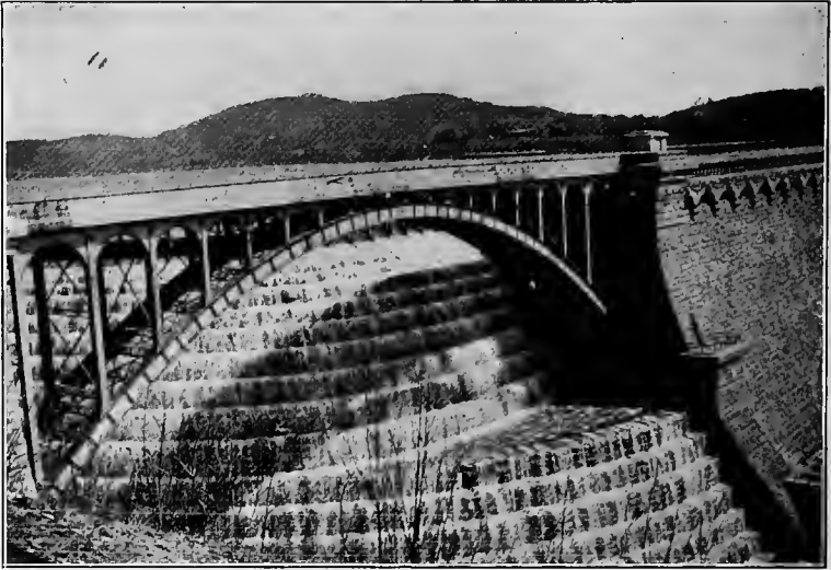
FIG. 63.—Spillway of the Croton Dam, Showing Natural Aeration.
