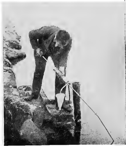
FIG. 9.—Plankton Pump. After Wilhelmi.
