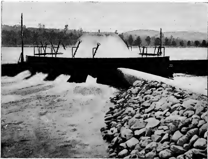
FIG. 66.—Aerator at the Ludlow Filter, Springfield, Mass.
