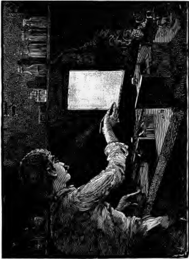
The Dark Room—coating the Plate.
