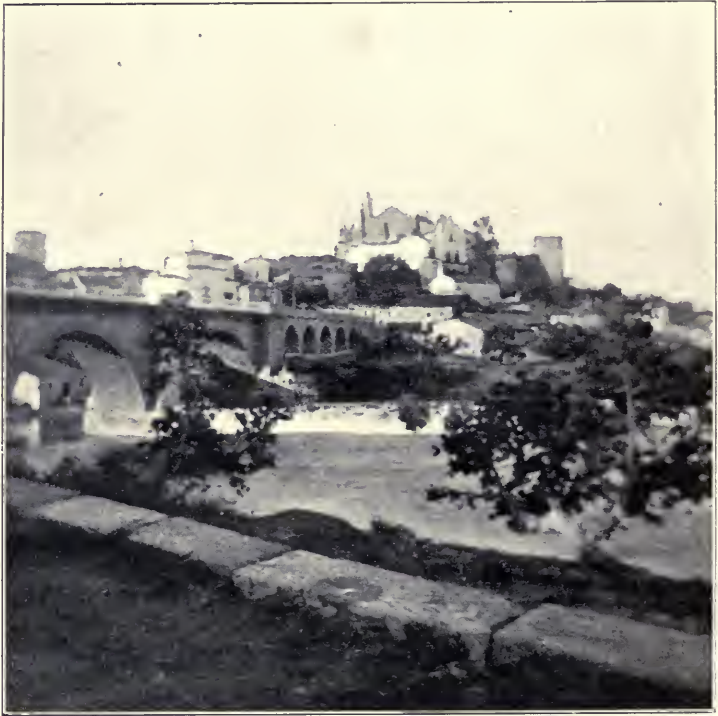
PLASENCIA, AND BRIDGE OVER THE RIVER JERTE.
