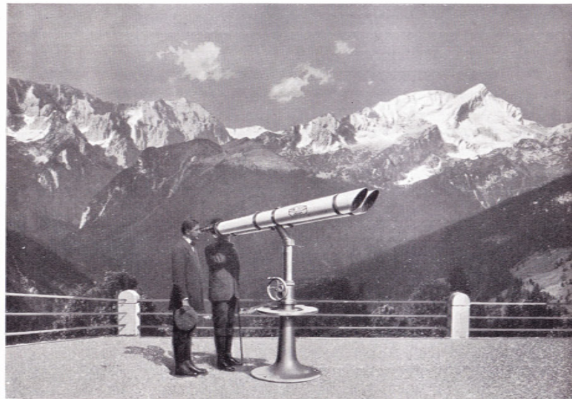
Fig. 27. Asal. Binocular Telescope on column used by two observers. 9195
