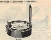
Liquid Prismatic Compasses. The liquid damps the oscillation of the compass ring and gives it a very smooth action. Made in two sizes.
